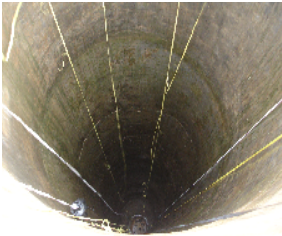
Photo 1: A water well
